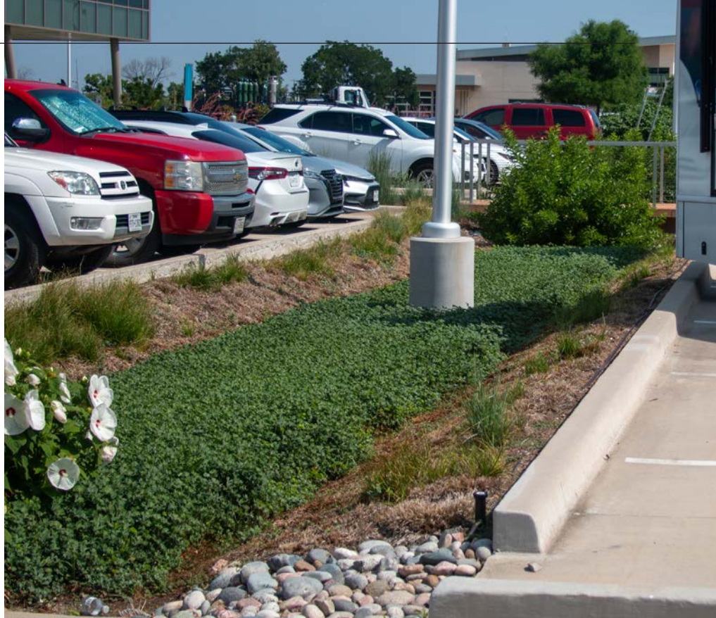
GSI practices in action at the Texas A&M AgriLife Research and Extension Center at Dallas: permeable pavement (left) and a bioswale depressed parking lot median (right). Photos by Leslie Lee, TWRI.
