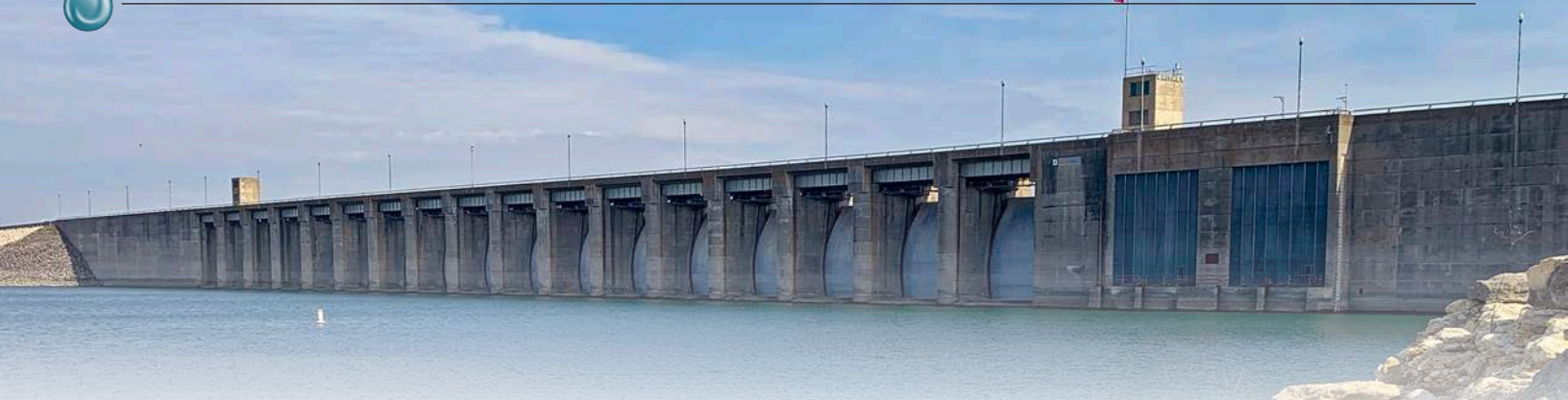
Whitney Lake Dam Gates (north side). Photo by Trevor Welsh, USACE.
